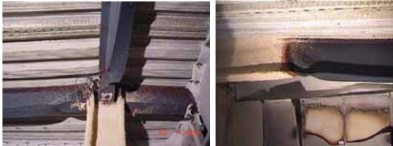
Figure 2.26 Various deformed steel beams
