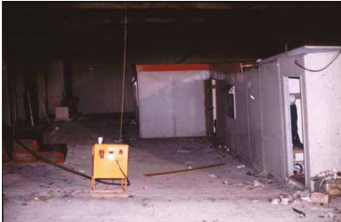
Figure 4.2 View of deformed floor above the fire (the maximum deflection was about 600 mm)
