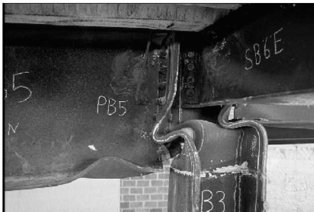
Figure 2.7 Squashed column head following the test
