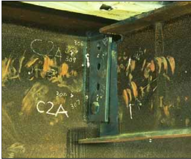
Figure 2.8 Fin-plate connection following test
