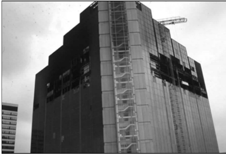
Figure 4.3 Churchill Plaza, Basingstoke following the fire
