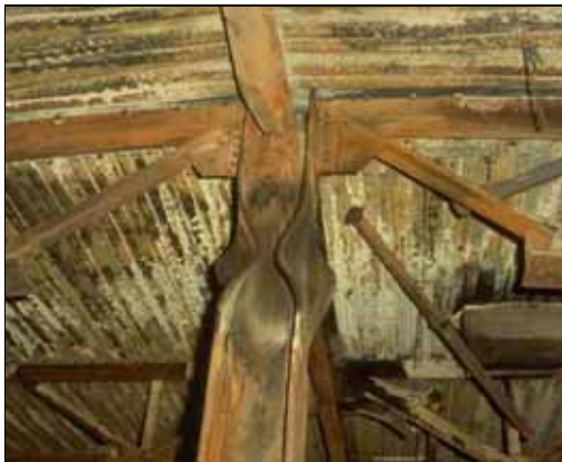
Figure 4.1 Buckled column and deformed beams at Broadgate
