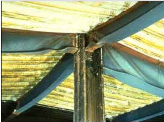
Figure 2.20 Column head showing buckled beams
