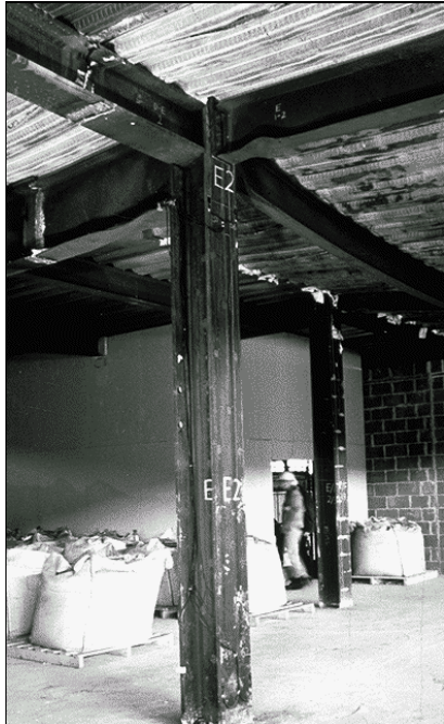
Figure 2.10 View of structure following test
