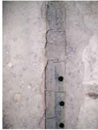
(b) State of the reinforcement joint at the location of the crack after cooling
