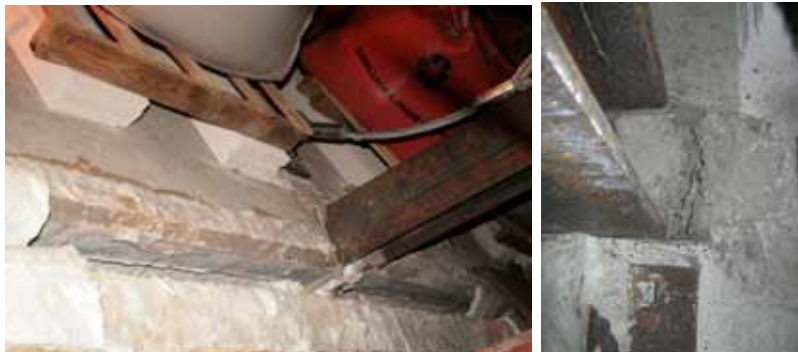
Figure 7.42 Cracking of concrete around central columns
