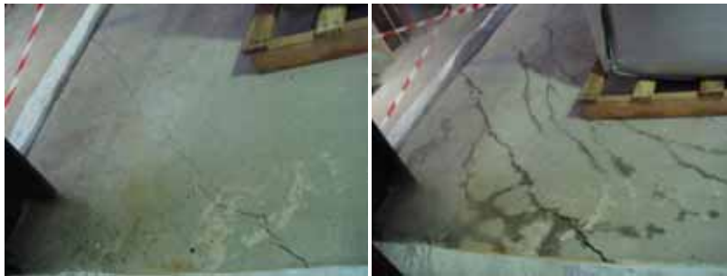
(a) At the beginning of fire test (b) At the end of fire test
