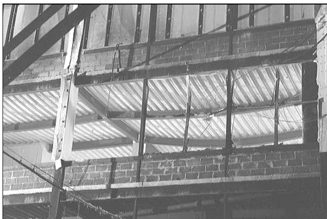
Figure 2.14 Deformed structure during fire
