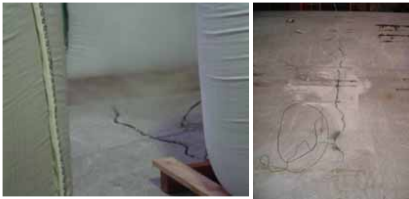
(a) State of the cracking at central part of the floor (b) State of the cracking after cooling
